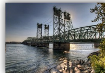
I-5 Interstate Bridge over Columbia River from Vancouver, WA
